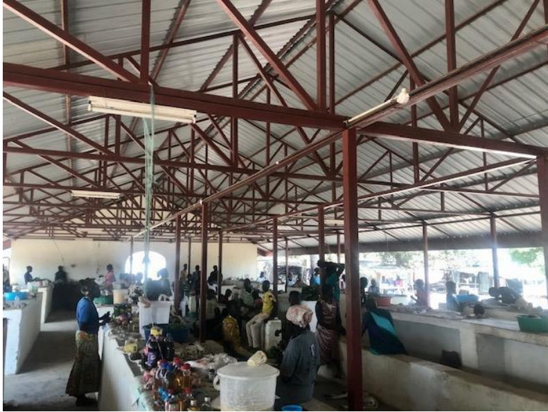
Wulu Market Shade, Lakes State- financed by the SAFER project
